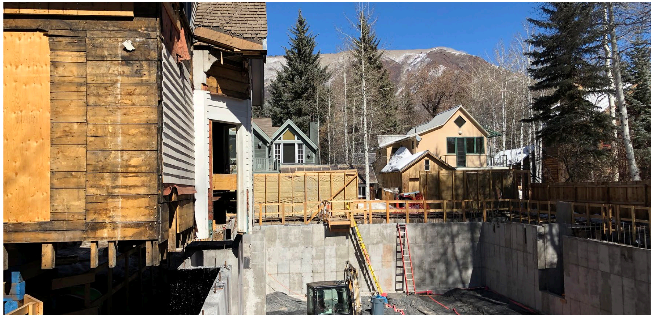
HISTORIC BUILDING RESTORATION
